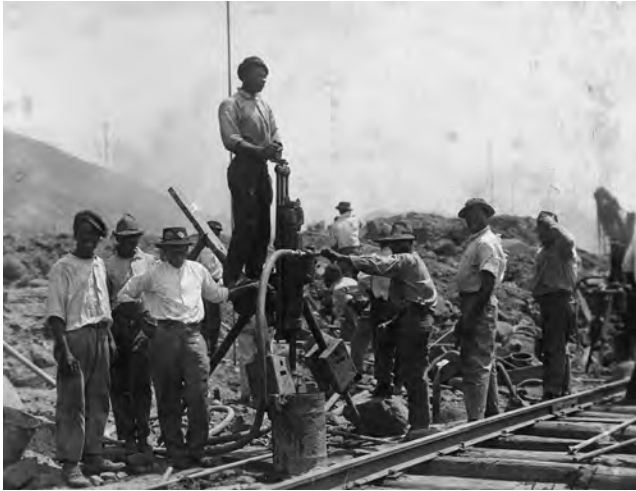
Railway workers with pneumatic drill. Undated photograph.
