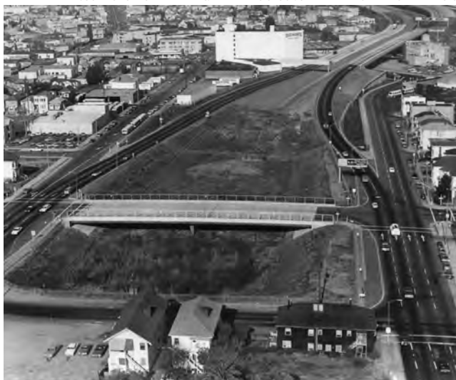
COURTESY OF ROY H. WILLIAMS/MEDIA NEWS GROUP/OAKLAND TRIBUNE VIA GETTY IMAGES Interstate 980 severed the predominantly Black neighborhoods of West Oakland from the rest of the city, setting the stage for underfunding of municipal projects in the area. Excavation site of Interstate 980. (1976)
